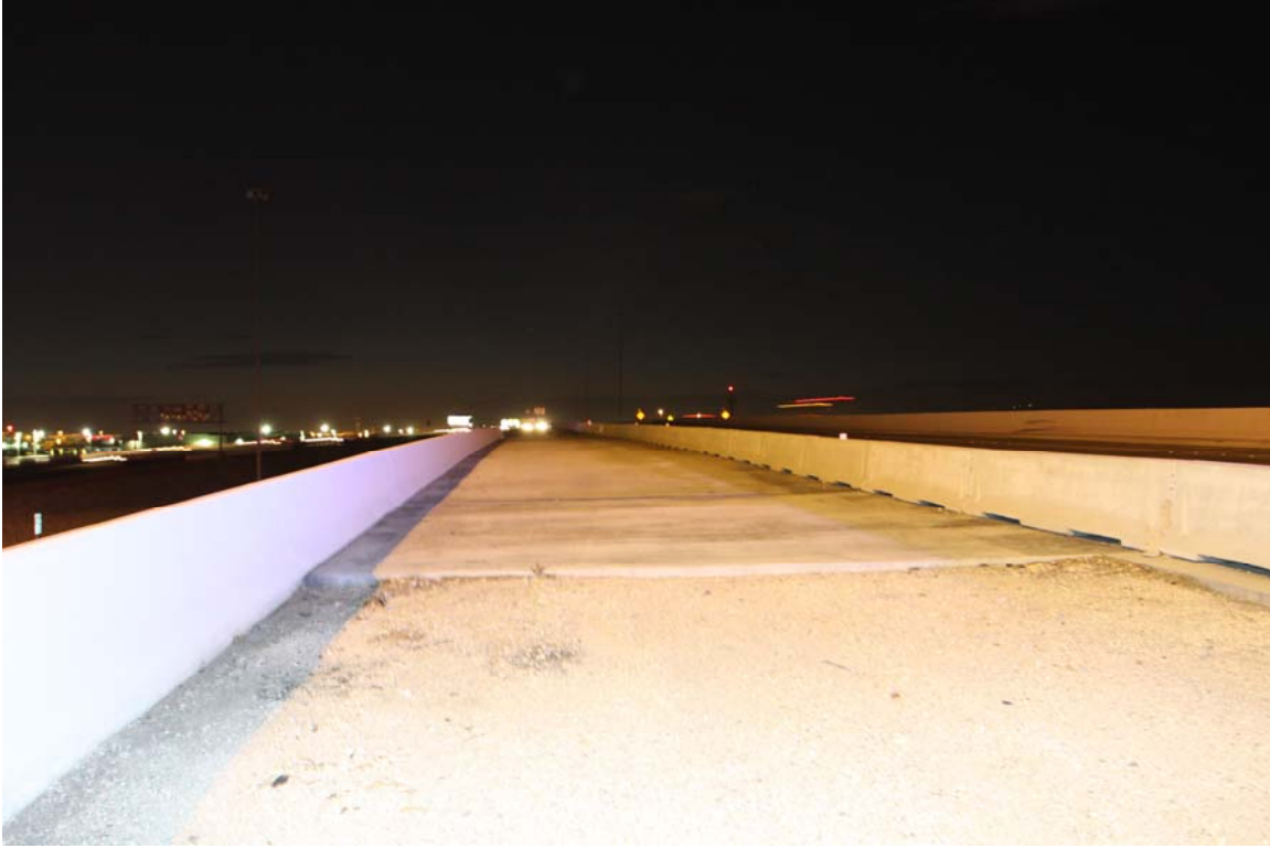
Construction access/extension bridge area on CC-215.
